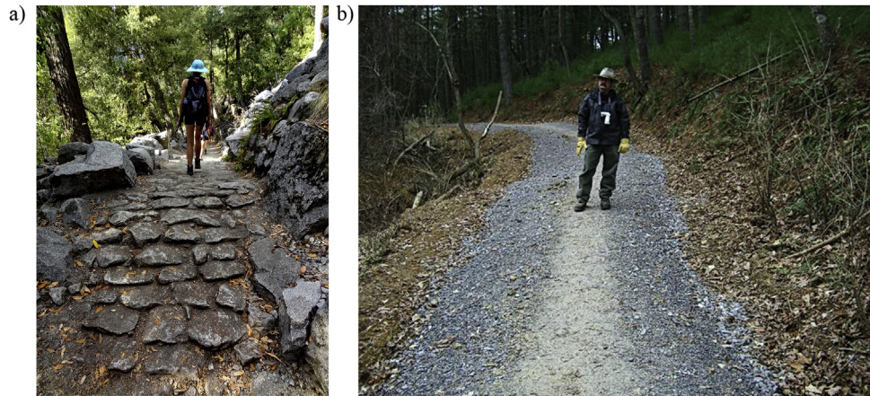
Fig. 4. a) Trails that must support heavy traffic, particularly by horses, can be armored with embedded rock (stone pitching). b) Crushed rock (gravel) also supports heavy traffic, though is more easily displaced when wet. Photos by Jeff Marion.
