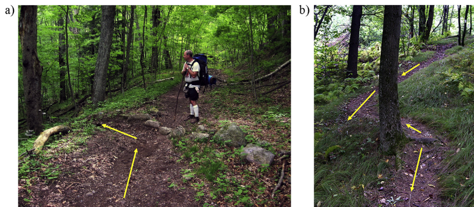
Fig. 3. a) This rock water bar is preceded by a ditch to drain water from the trail. b) Grade-reversals temporarily reverse the grade of the trail so that all water drains off; these rarely require maintenance. Photos by Jeff Marion.
