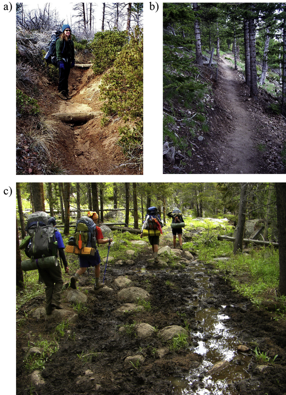
Fig. 2. a) Steep fall-line trails (TSA <math><22^\circ</math>) erode rapidly. b) Side-hill contour-aligned trails (TSA >math>>69^\circ</math>) resist widening, muddiness, and soil loss. c) TSA is less influential in flat terrain where trail widening and muddiness are common problems. Photos by Jeff Marion.
